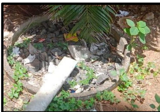
Rainwater harvesting units in MAMSE, Tiruchirappalli, Tamilnadu.
