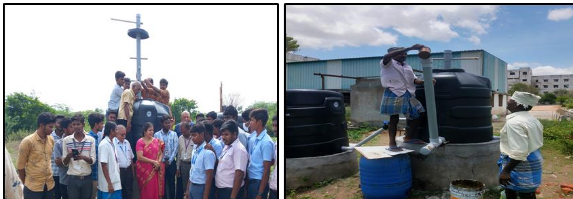
Biogas Plant Facility at MAMSE, Tiruchirappalli, Tamilnadu.
