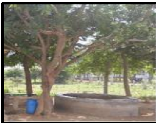
Composting unit at MAMSE, Tiruchirappalli, Tamilnadu.
